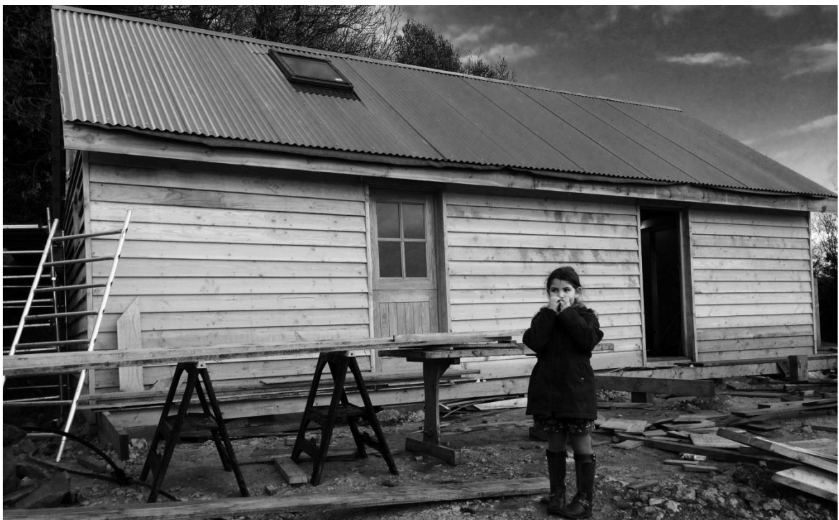
(The new barn being constructed)
