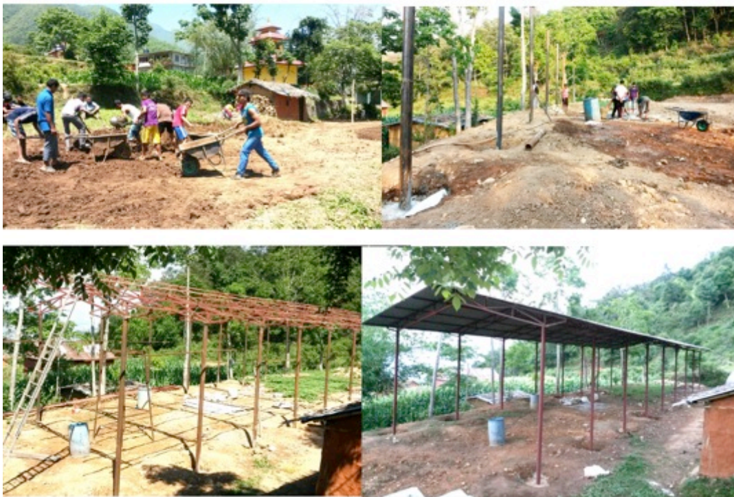
Constructing a temporary shade as a replacement of the severely damaged cowshed-dormitory complex.
