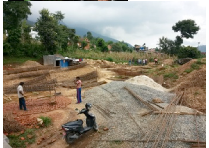
New school building under construction
